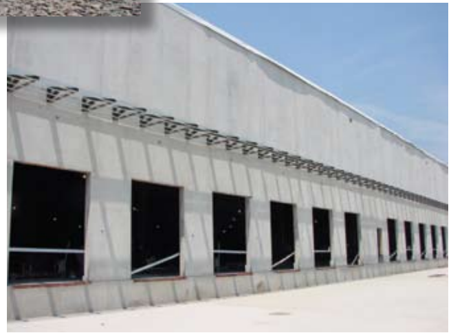
Use of insulated wall panels contributed to achieving LEED points for the Anheuser-Busch Distribution Center. These included supplementary points under the Energy & Atmosphere category as well as points for diverting construction waste, using recycled materials, and using locally obtained materials.
