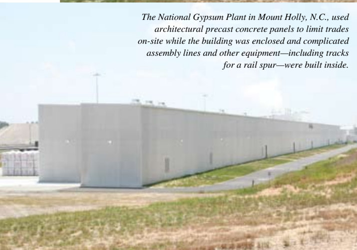
The precast concrete panels on the National Gypsum Plant feature exposed aggregate that was sand-blasted in the field and left unpainted. The smooth panels don't allow dust to collect, a key concern for manufacturing plants.
