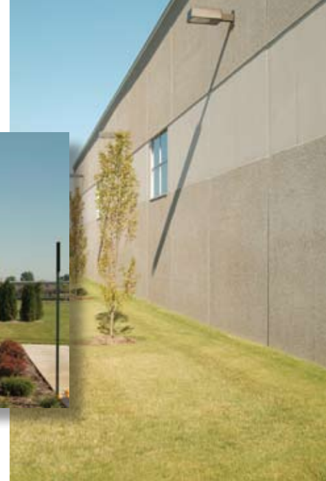
Action Packaging in Caledonia, Mich., used precast concrete wall panels with 2 in. of insulation sandwiched between two 3-in.-thick wythes of concrete to speed construction while providing an energy-efficient design.
