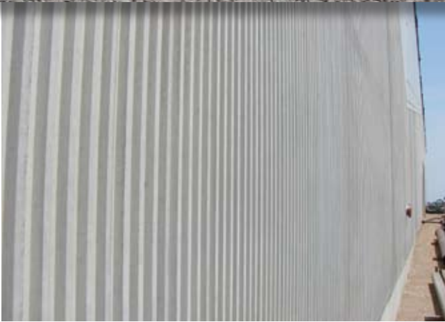
Use of insulated wall panels contributed to achieving LEED points for the Anheuser-Busch Distribution Center. These included supplementary points under the Energy & Atmosphere category as well as points for diverting construction waste, using recycled materials, and using locally obtained materials.
